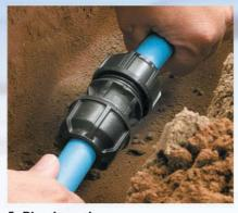
Pipe insertionSlide the pipe fully into the fitting to the point where the stop is felt.
